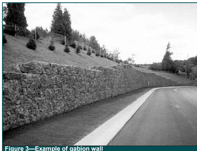
Figure 3—Example of gabion wall
